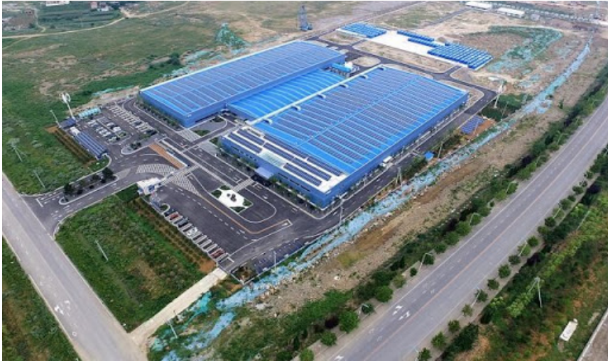
Dalian site China, 200 MW/800 MWh
