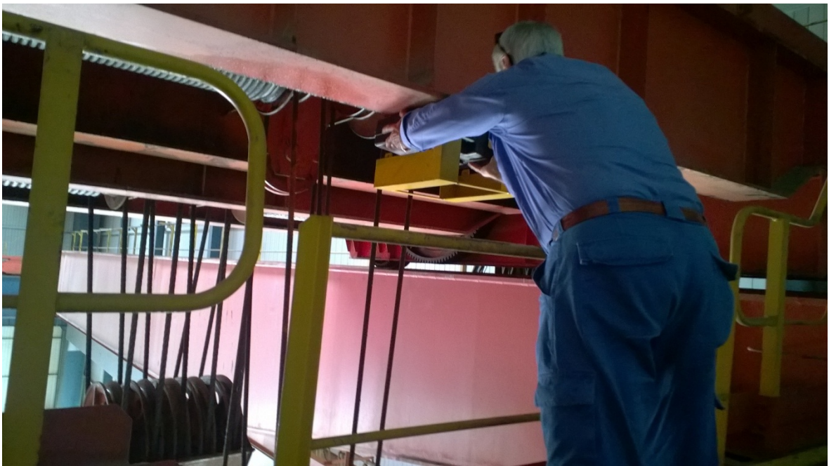
Figure 22. Installation of the prototype by the crane-operator.
