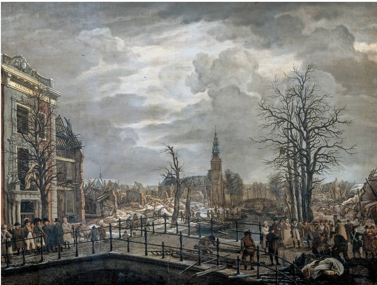
FIGURE 7 NOT FORGETTING: CAREL LODEWIJK HANSEN - RAPENBURG, LEIDEN 1807 AFTER THE EXPLOSION OF A GUNPOWDER SHIP ON 12 JANUARY 1807, WITH LOUIS NAPOLEAN BONAPARTE INSPECTING THE DAMAGE ON THE LEFT (RIJKSMUSEUM)..
